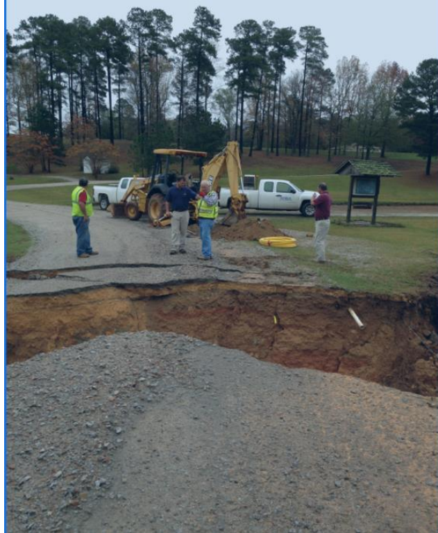
Fig. 3 -15 Fish Hatchery Road November 2015 (Hanging Rock Creek) Road failure due to extreme wash downstream from an earthen dam.
