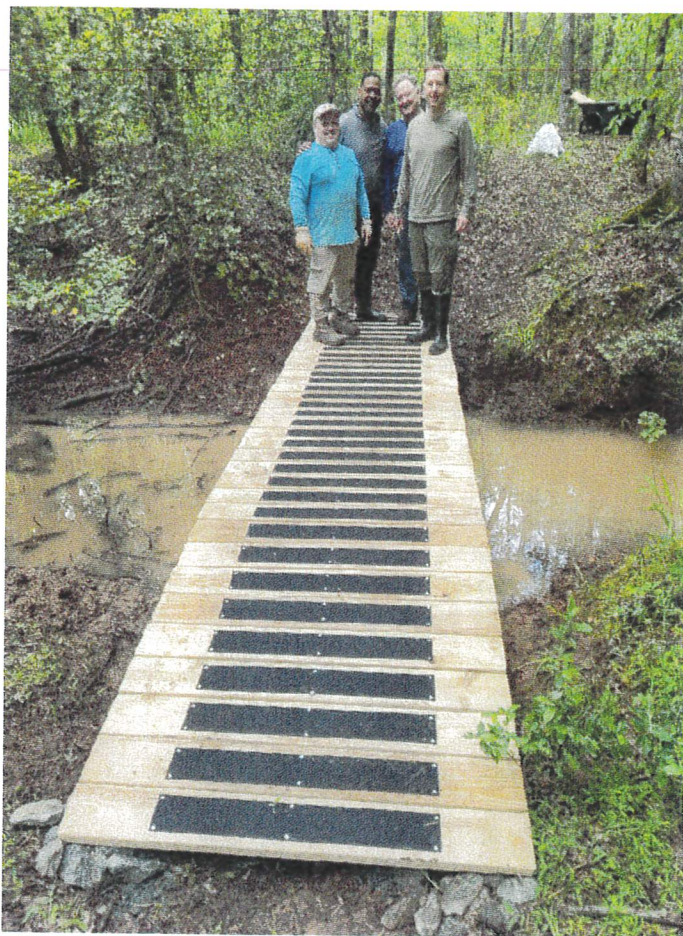
18' bridge over creek on new ½ mile trail extension along the Catawba from the picnic tables south to Waxhaw Creek. Front step has since been ramped and steps built up the slope in the back.
